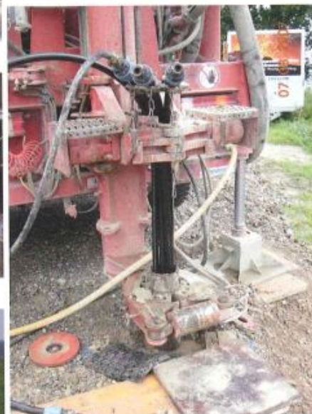
Figure 7. During grouting the auxiliary casing still prevents the borehole from collapsing. The BHE is under pressure (picture: Polydynamics Engineering Zurich)
